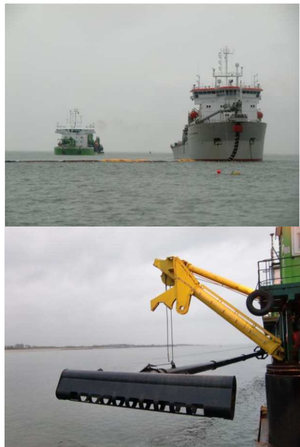
Figure 6. TSHD connected to floating line (above) and detail of diffuser head (below).
